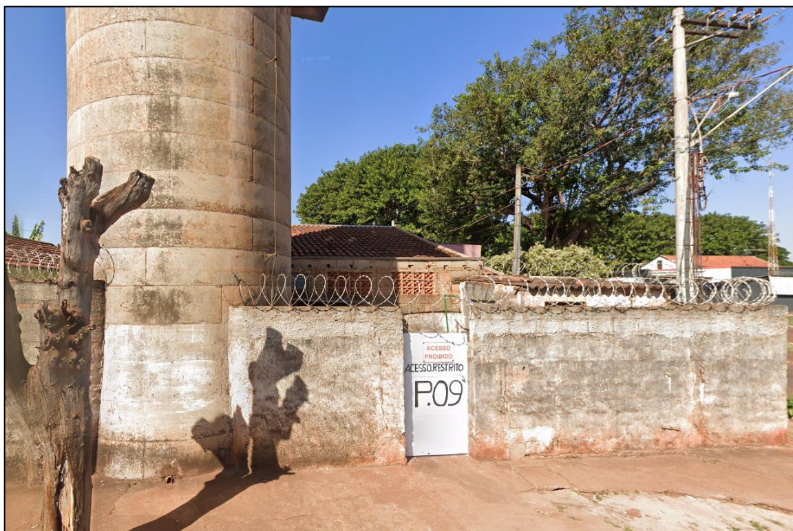
Figura 27 – Poço P 09 – Rua José Leonel Pupo, s/n.
