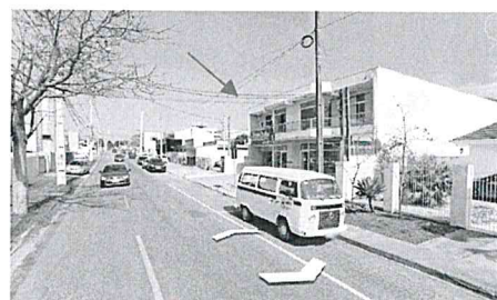
Fig.06: Imóvel 051.047.0386 (Google Earth)
